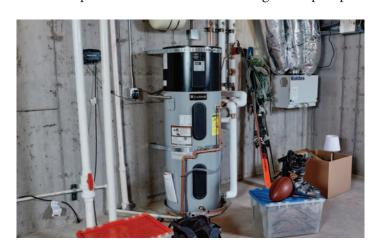
By moving heat instead of creating it, a heat pump water heater uses 60% less energy than electric storage water heaters. Photo Credit: Hot Water Solutions
