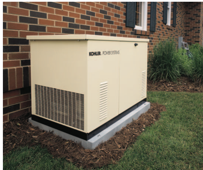
Left: If you purchase a portable backup generator, protect your home and family by taking the time to read the manufacturer's instructions. Photograph by Honda Above: Standby generators are permanently wired into the home's electrical system by a qualified electrician. Photograph by Kohler
