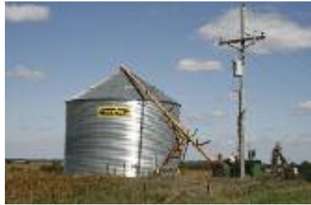
Watch for overhead obstructions and electrical wires. Electrocution can occur without direct contact.
