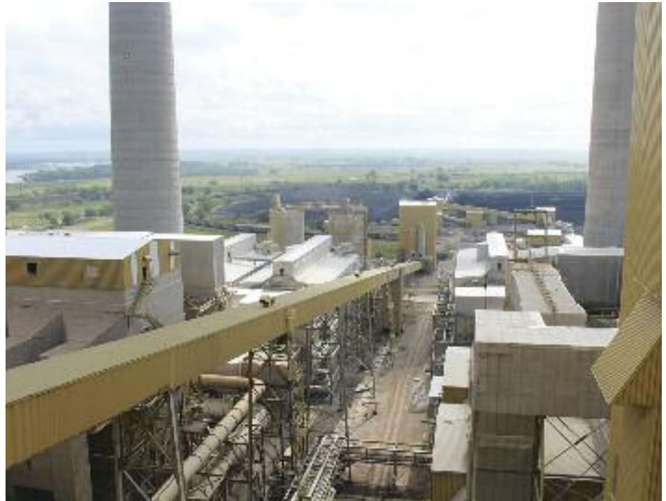
Gerald Gentleman Station (GGS) is Nebraska's largest generating plant. Located near Sutherland, Neb., the plant consists of two coal-fired generating units, which together have the capability to generate 1,365 megawatts of power.
